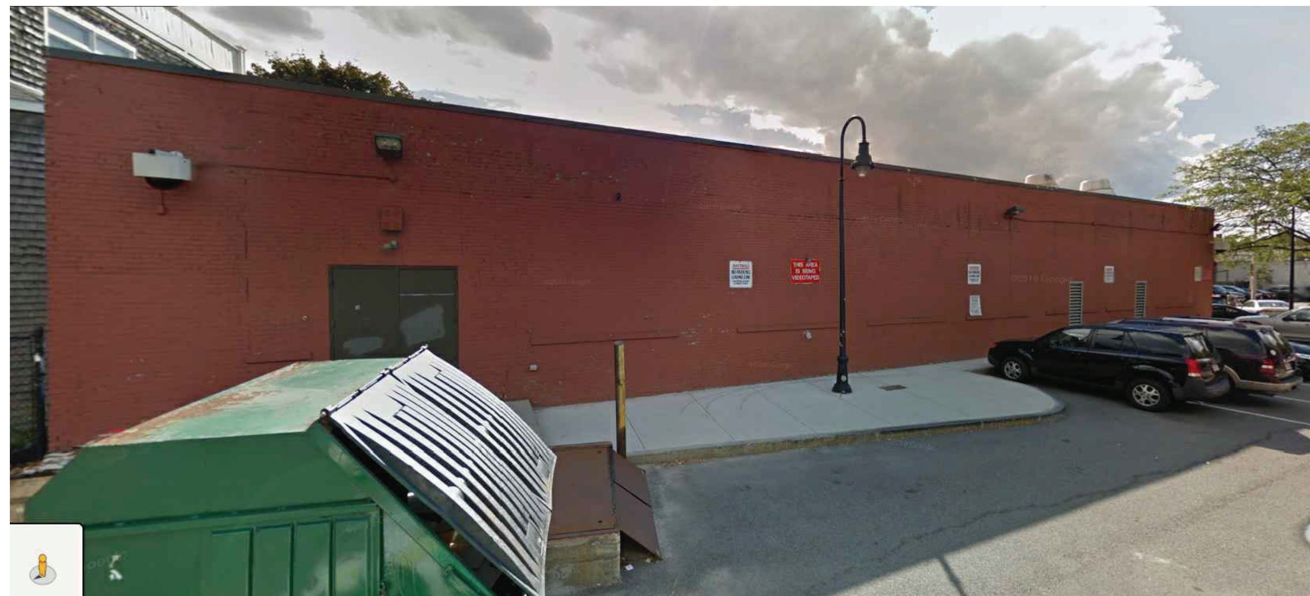
5 VIEW AT REAR LOADING AREA
